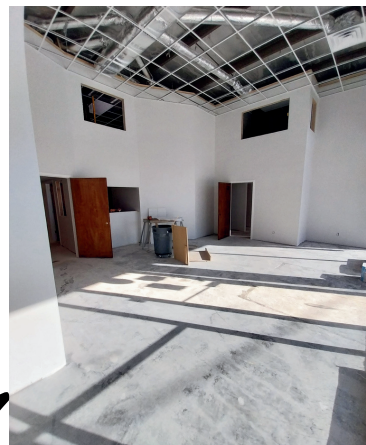
The RPS front lobby approaching completion!
